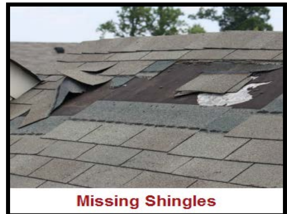
A Condition where Water would Enter
