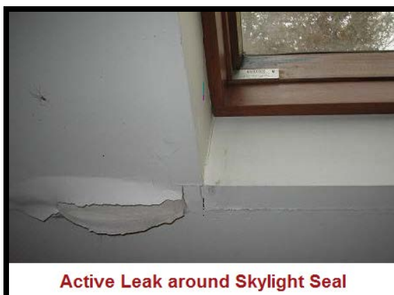
Visible Water Intrusion from Rain
