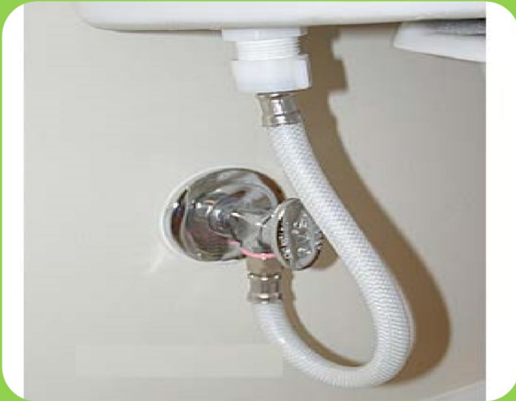
Line Appears Intact
