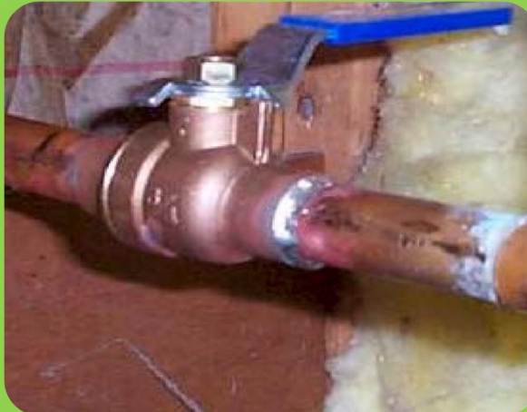
Valve Appears Intact
