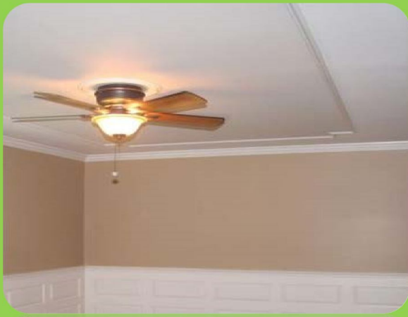
Ceiling and Walls are Dry
