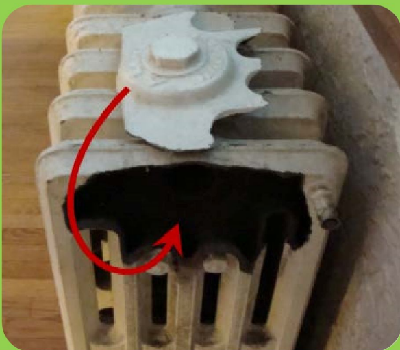
Freeze: Section of Radiator Broken
