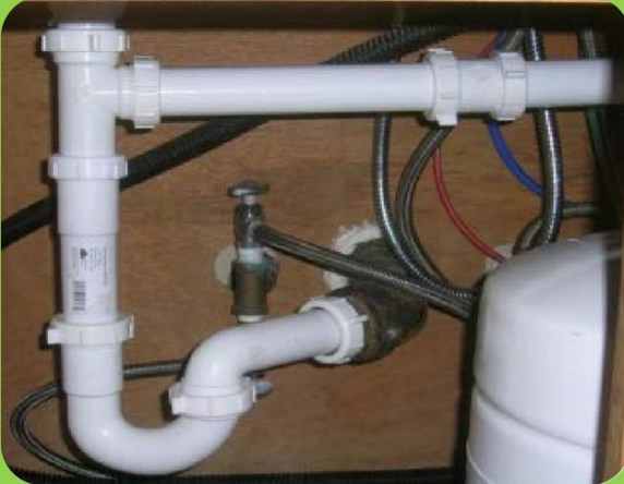
Joints Appear Intact
