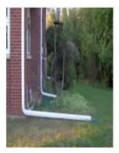
This is an example of an excessive extension. The extension should be cut to the appropriate length
