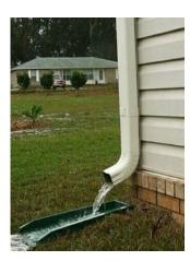
Splash pad is diverting water away from the foundation and protecting the ground from eroding causing a hole or damage to the landscape
