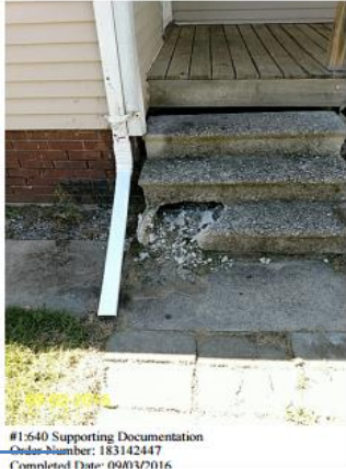
This is incorrect
