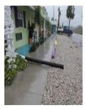
This is an example of a trip hazard being created by installing the downspout extension
