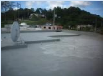
11/27/11 Roof was initially repaired
