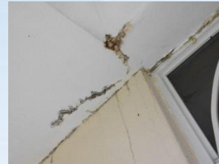
Water damage originally reported worsened over time with new/additional damage going unreported (09/30/11 to 05/19/12 to HPIR)
