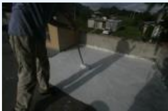
12/5/12 Roof patched again
