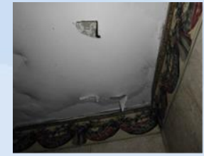
Water damage originally reported worsened over time with new/additional damage going unreported (09/30/11 to 05/19/12 to HPIR)
