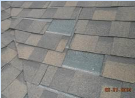
Missing Shingles
